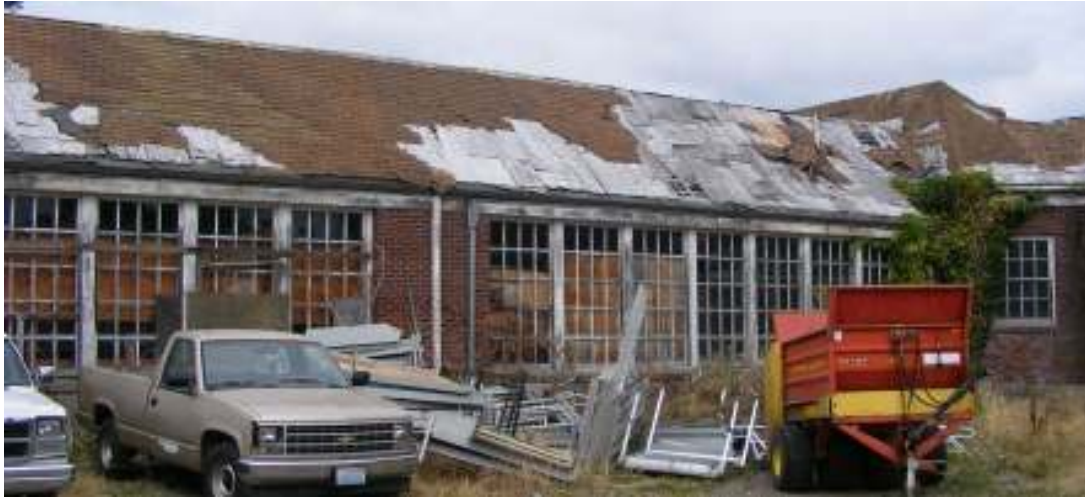
Central School building in 2011 photo from rear (west side) looking northeast.
