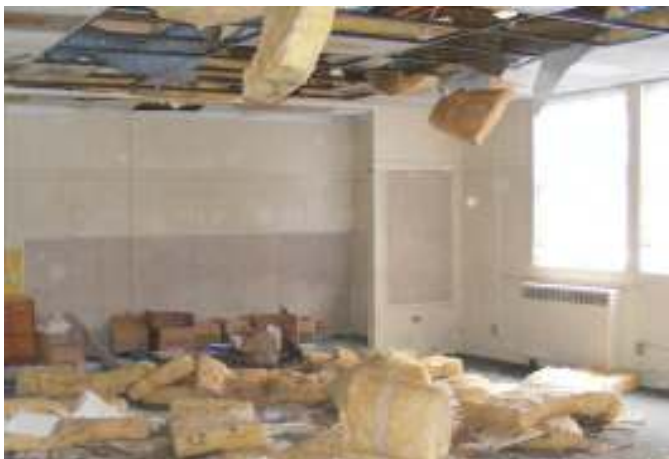
Central School interior, October 2011
