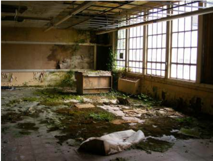
Central School interior, October 2011
